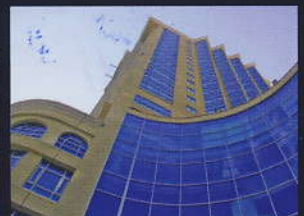
Hotel Resort Project
